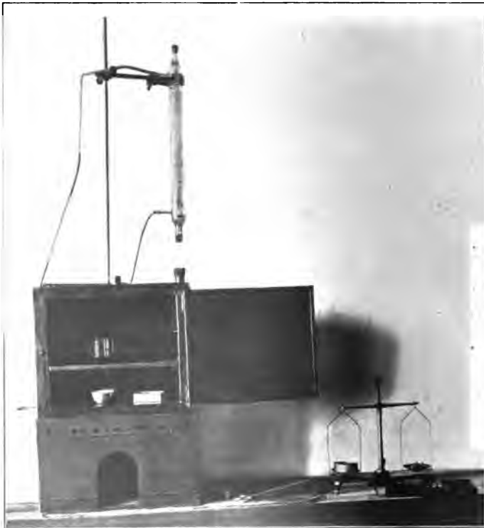
FIG. 52. Apparatus for determining Moisture Content of Soils.
